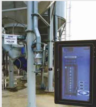
Automatic control system Silotouch including touchscreen, pressure switch, control panel and sleeve valves.
