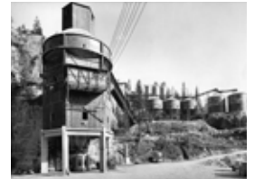
The first plant supplied by CIFA in 1956 with 300 m 3 /h output capacity for Alpe Gera DAM project (Italy)
